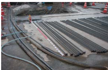
写真-3 Post-Head-Bar
